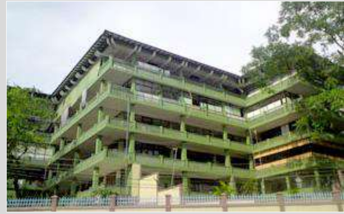
NORTH COLOMBO MEDICAL HOSPITAL - RAGAMA
