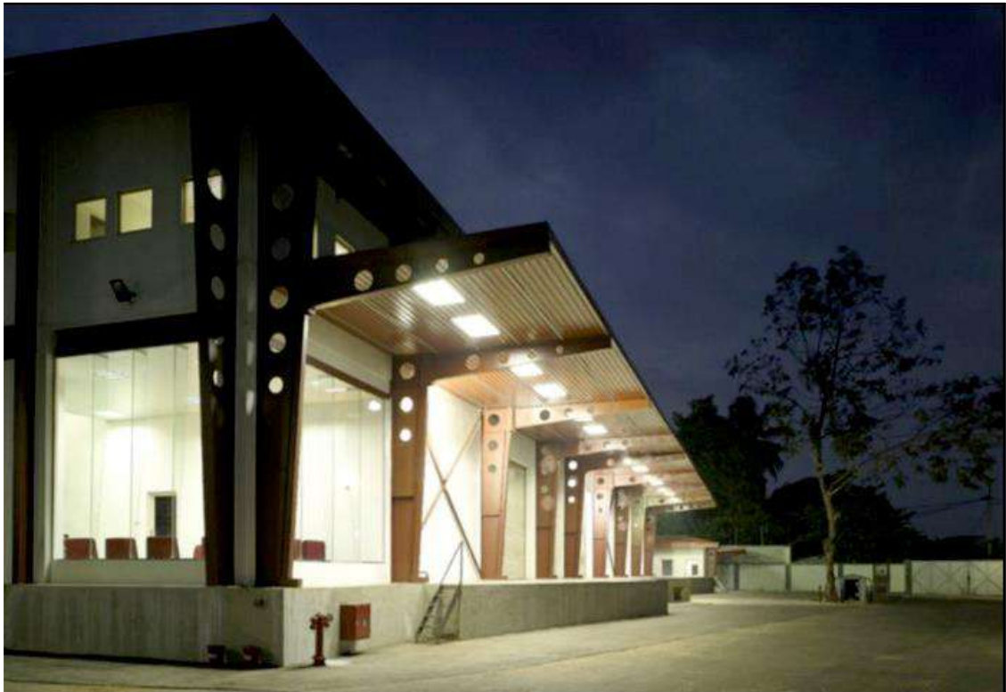
WAREHOUSE AT SEEDUWA FOR (DSCL)
